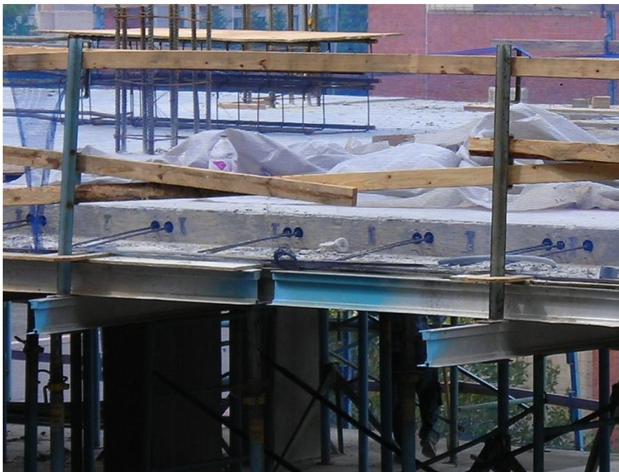
*Photo 11: View of post-tensioning cables prior to jacking force application.*
