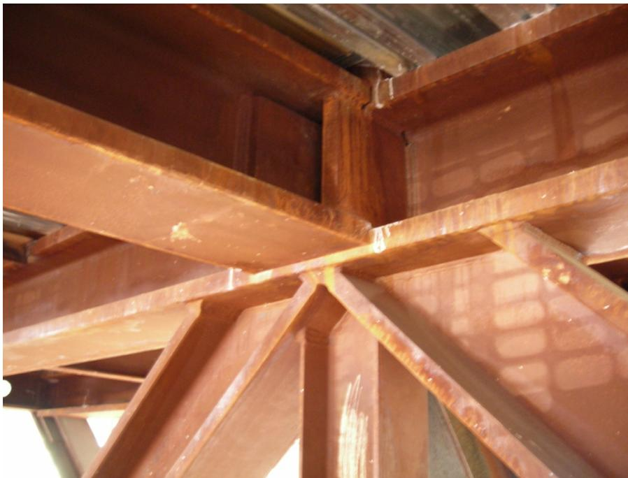
*Photo 9: Typical full penetration welded connection of the bridge truss structure.*
